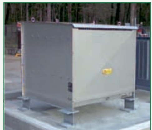
2*770 Ohm, 90s, 11.55 kV luftgekühlt
